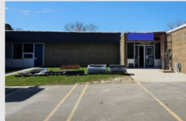
Exterior door, glazing, & panel replacement
