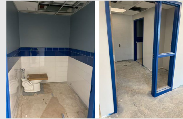
Toilet Room at Clinic
