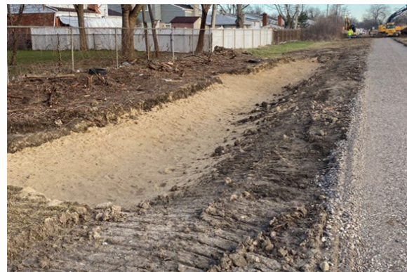
Site improvement - bioswale
