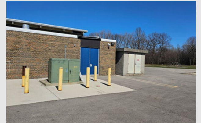
Exterior door and panel replacement
