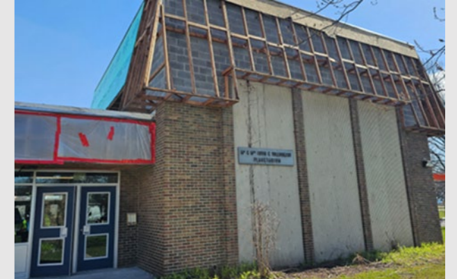
Removal of exterior stone panels
