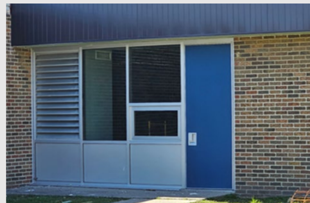
New exterior doors, glazing, and louvers
