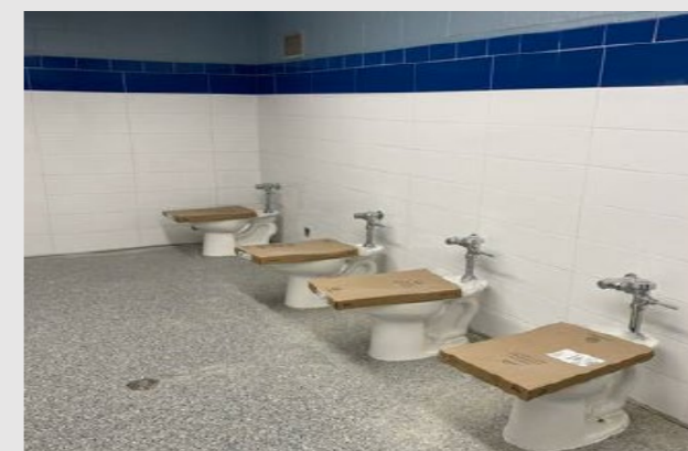
Multi Stall - Toilet Room renovation
