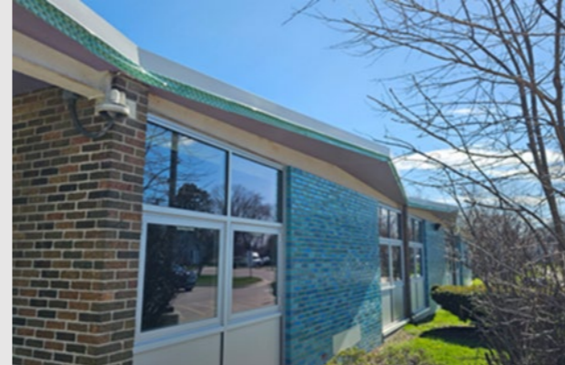
New exterior glazing
