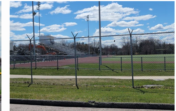
Bleacher demolition @ University K-12 / MacArthur K-8 Campus
