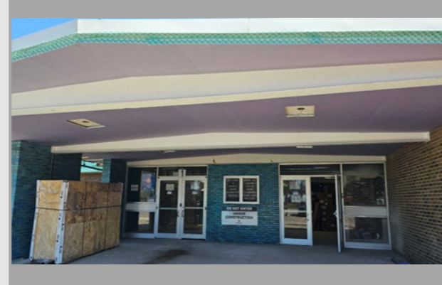
Main entry canopy soffit replacement
