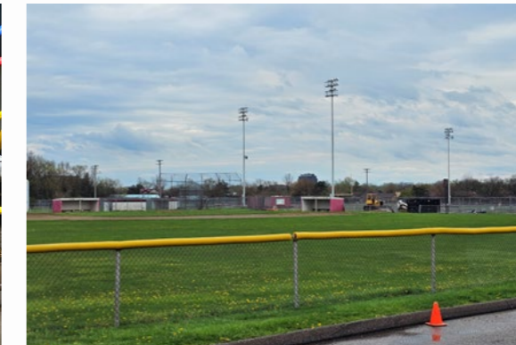
Bleacher demolition @ University K-12 / MacArthur K-8 Campus
