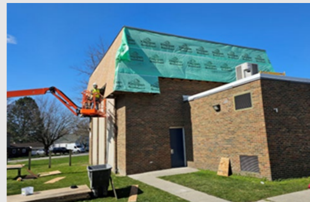
Exterior sheathing installation
