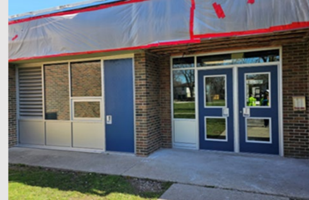
New exterior glazing, louvers, & doors
